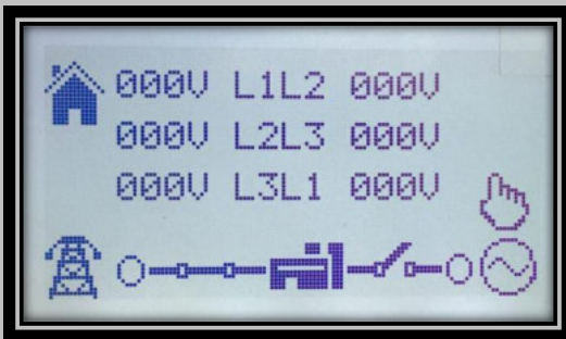
Generator & Mains Voltage (L-L)
